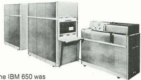
The IBM 650 was a widely used general-purpose computer for business, industry, and universities. When introduced, it processed data on punched cards. Later users could add magnetic tapes and disks. The 650 had a magnetic drum memory.
